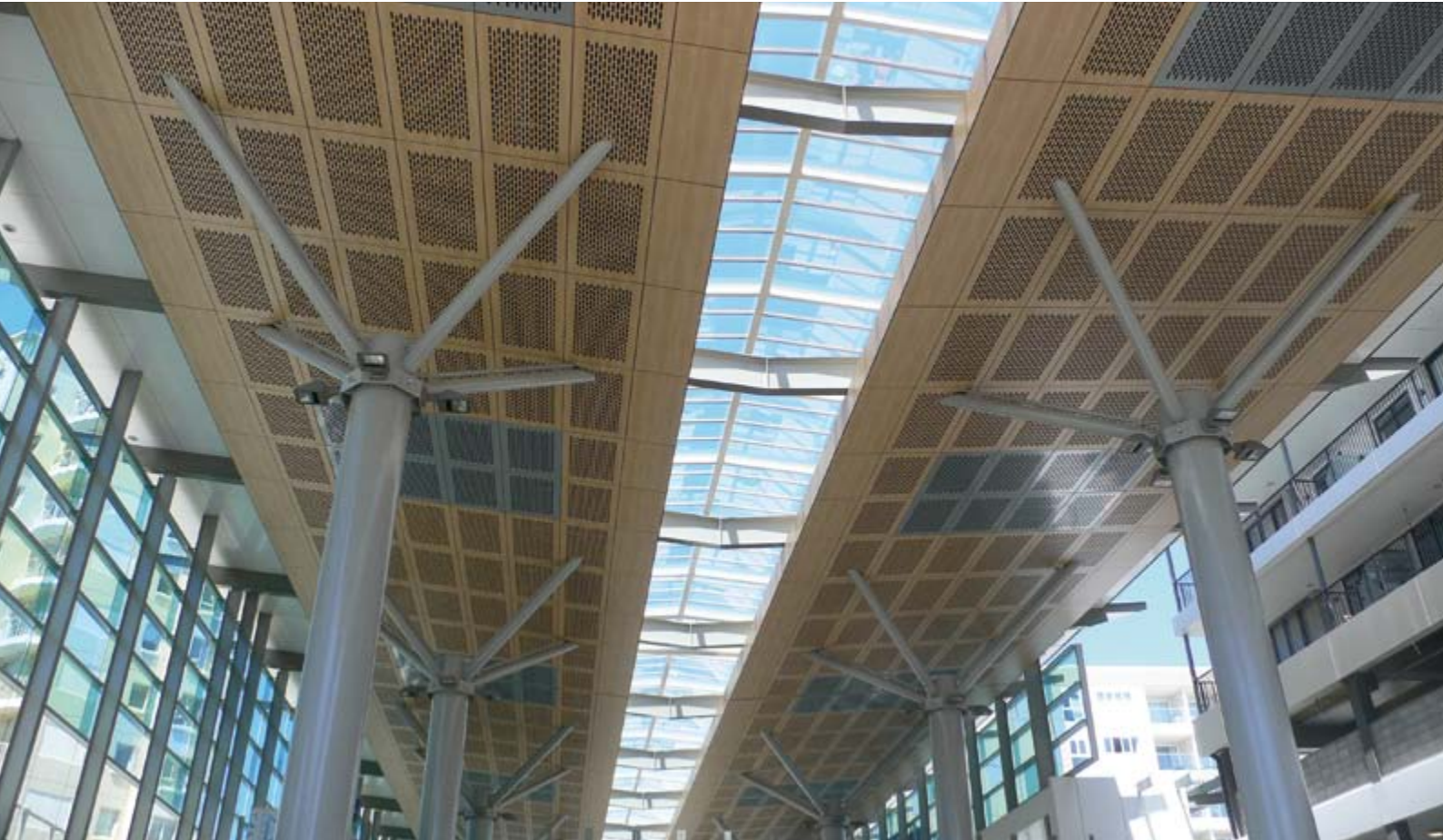
Project _Newmarket Railway Station, Auckland Country _New Zealand Design _Opus International Consultants Ltd. Images _John Gibbons Decor _0125 NT
