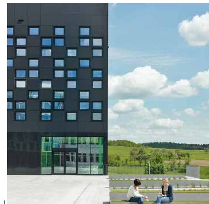
1-2 Office and Conference Centre, Heroldsberg, Germany, A+D 48 mv architect + starkearchitektur, Köln (Photos: Paul Ott)
