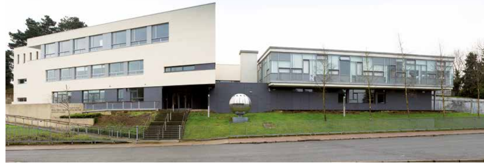
2013, New extension on top of the 2006 extension. The plinth to the right and left of the entrance is clad with the same dark coloured fibre cement panels and provides a visual link between the two buildings.
