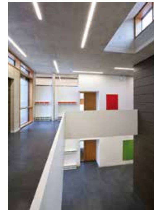
Interior walls are partly clad with fibre cements panels as well.
