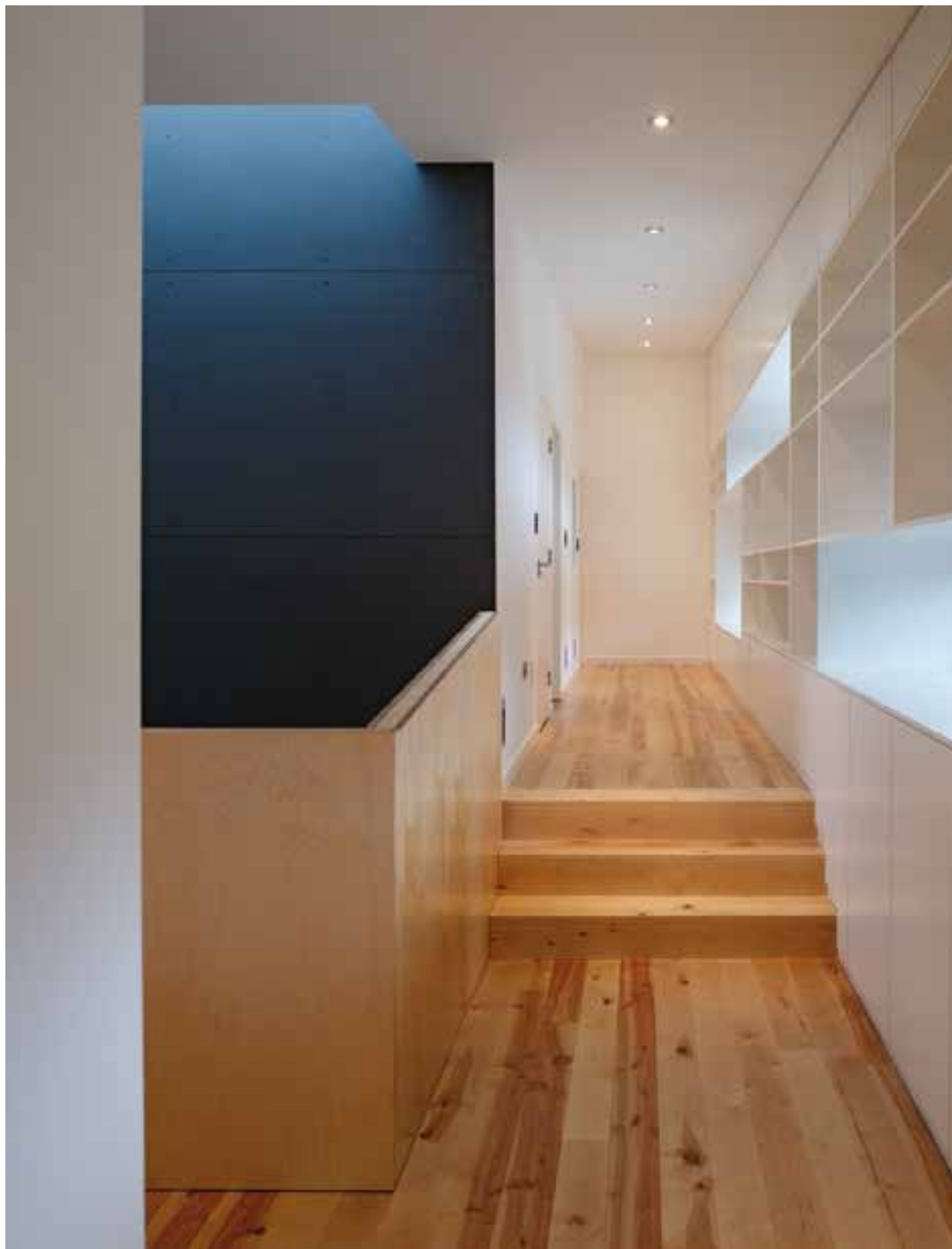
Upper floor, view of the hallway looking south The staircase wall is clad with the same fibre cement panels as the façades.
