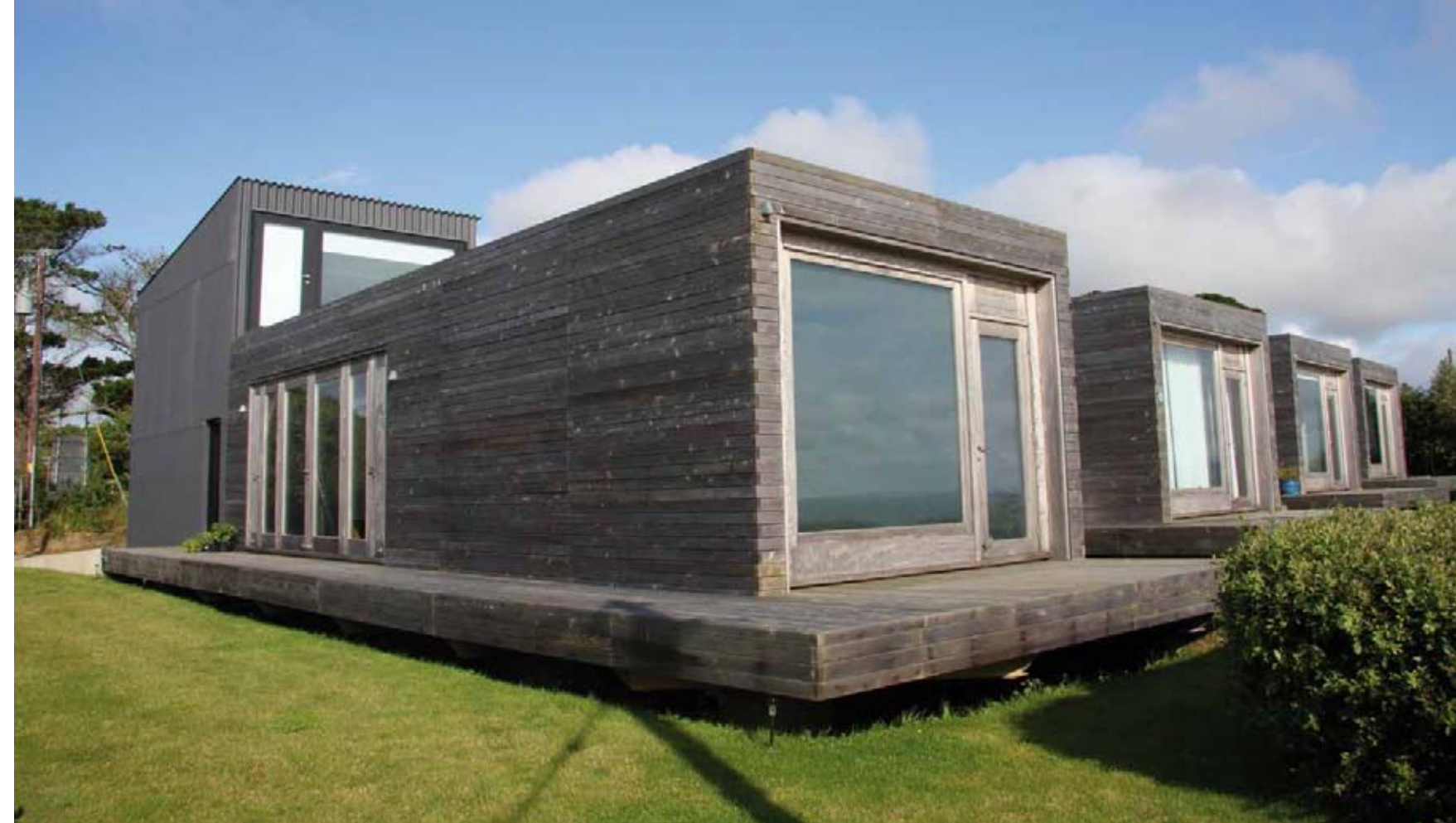
Corrugated fibre cement sheets and cedar determine the exterior appearance of the four identical houses.
